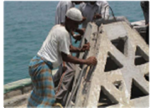
Pyramid shaped locally-made structure for rehabilitation coral reefs in Salakh
